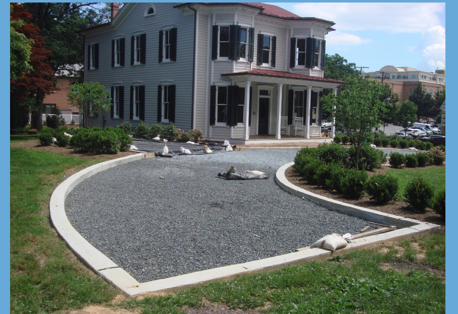
An historic house on West Jefferson Street installed a permeable paver driveway in 2018, shown here during construction of the gravel subsurface.
