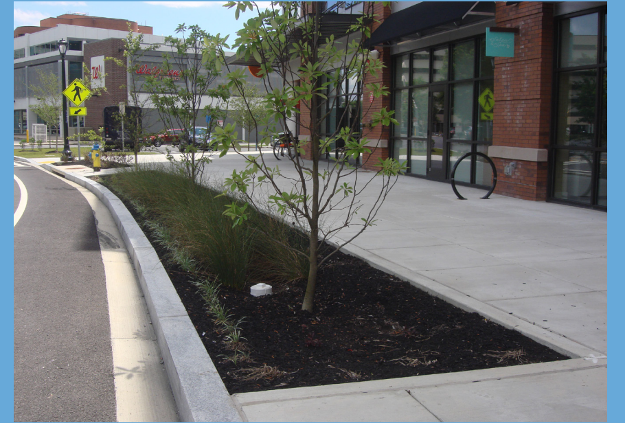
Bio-retention landscaping was installed between the sidewalk and street curb as part of new development along Dawson Avenue.
